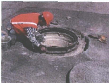
FIGURE 3-1 Sewer Manhole Installation
